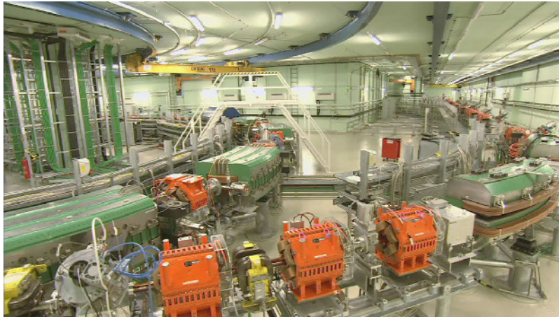
Figure 3.5: picture of some of the MAPTA components taken at the beam extraction section. It is possible to see part of the synchrotron (left side) and of the HEBT (right side). The dipoles and quadrupoles are colored in green and orange respectively.
